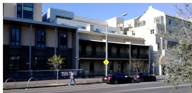
210-214 Leicester Street [216 demolished]
