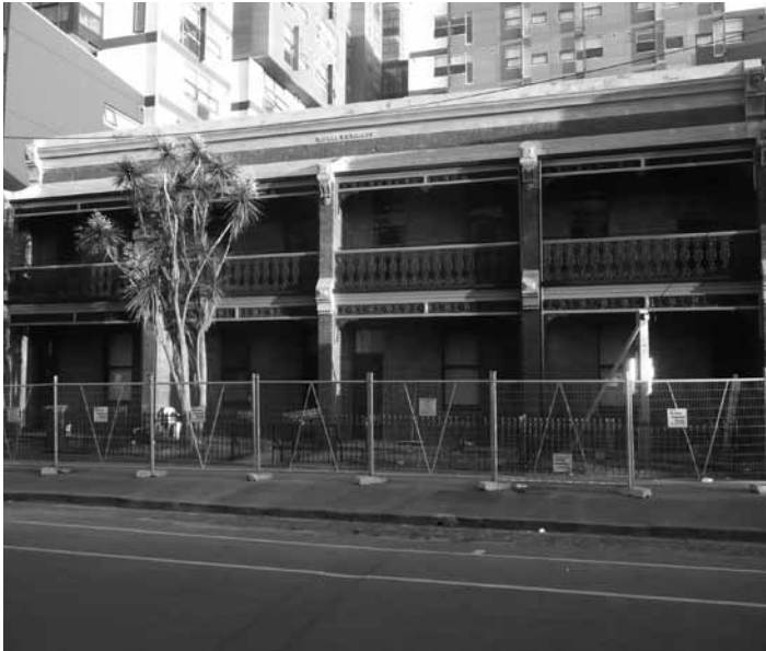
Restoration work being done on Royal Terrace in Faraday Street
