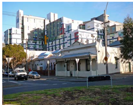
Terrace houses (Faraday St. with Eastern Precinct backdrop) saved by CRA through VCAT action against Melbourne University demolition plans
