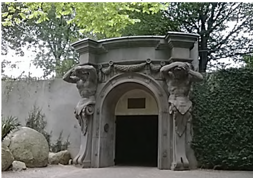
Image 3: Colonial Bank Door [Entry to Underground Carpark]
