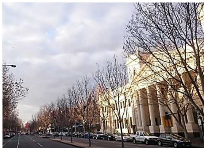
The Trades Hall Building – not a significant streetscape?
