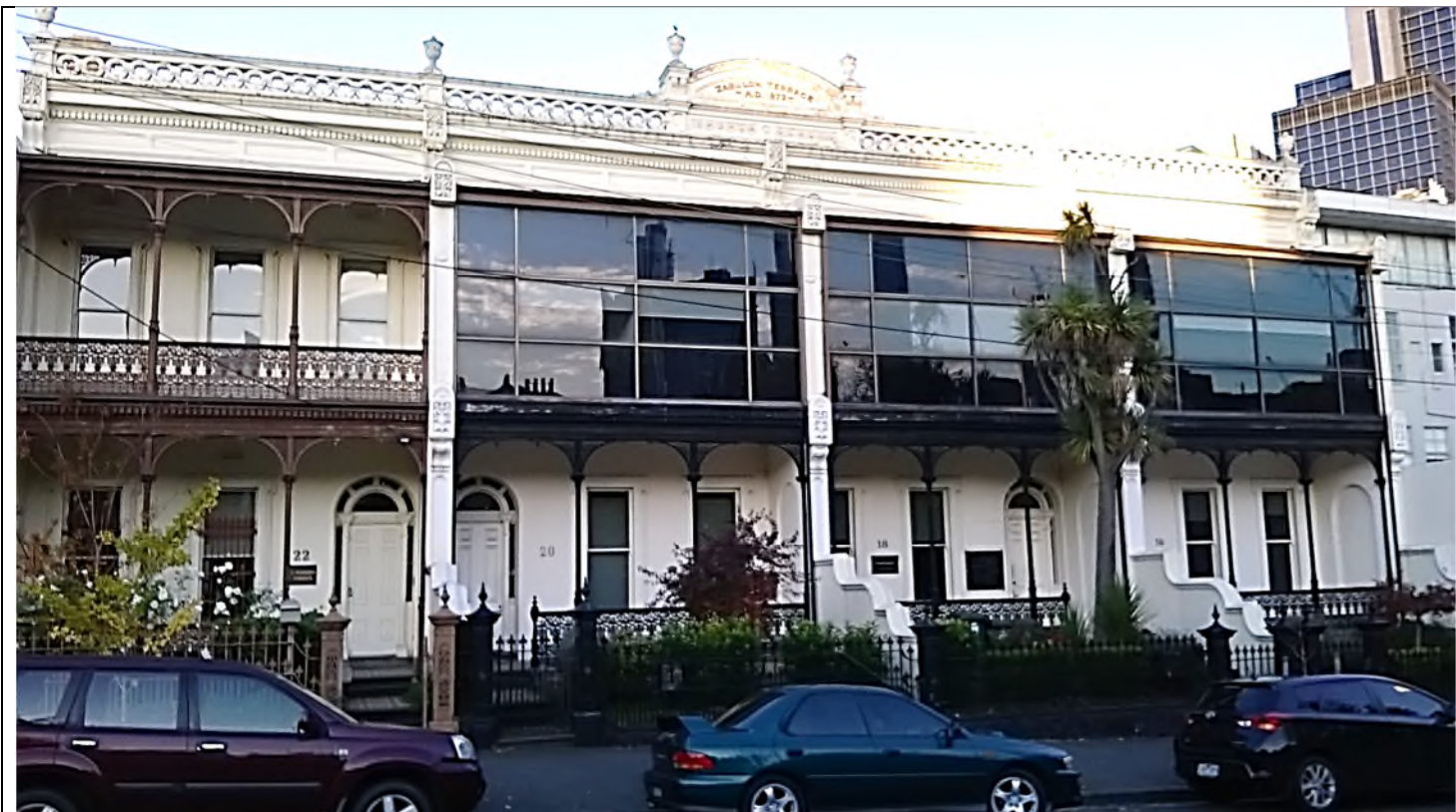
16-22 Drummond Street Carlton – Existing Condition
