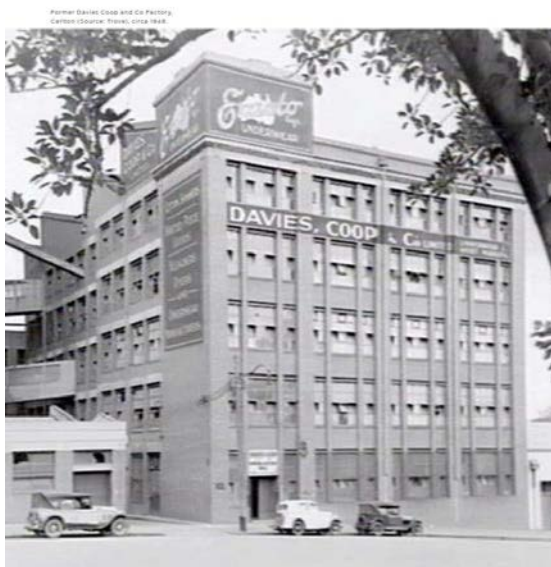
Figure 7. c1930s. From HIS page 9, showing hopper windows broadly consistent with 1927 drawings. Original entry form also evident. (From application documents)
