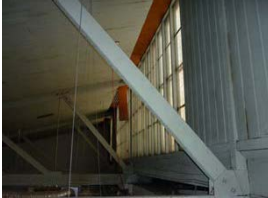
Figure 3. Saw tooth roof internal view of south glazing and timber trusses. (M.Gould 2015)
