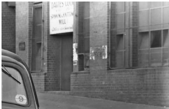
Figure 7. c1930s. From HIS page 9, showing hopper windows broadly consistent with 1927 drawings. Original entry form also evident. (From application documents)
