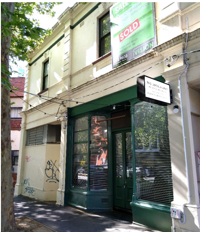
138 Queensberry Street following refurbishment [Image taken December 2021 E. Ogilvy]
