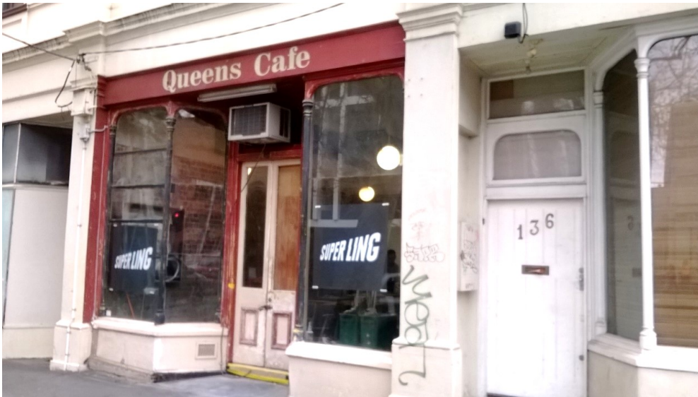
138 Queensberry Street before refurbishment
